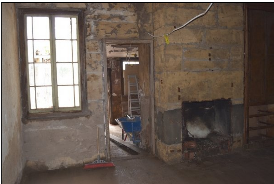
BEFORE: Layers of wallpaper and plaster had to be removed and damp walls dried out as part of the renovation.
