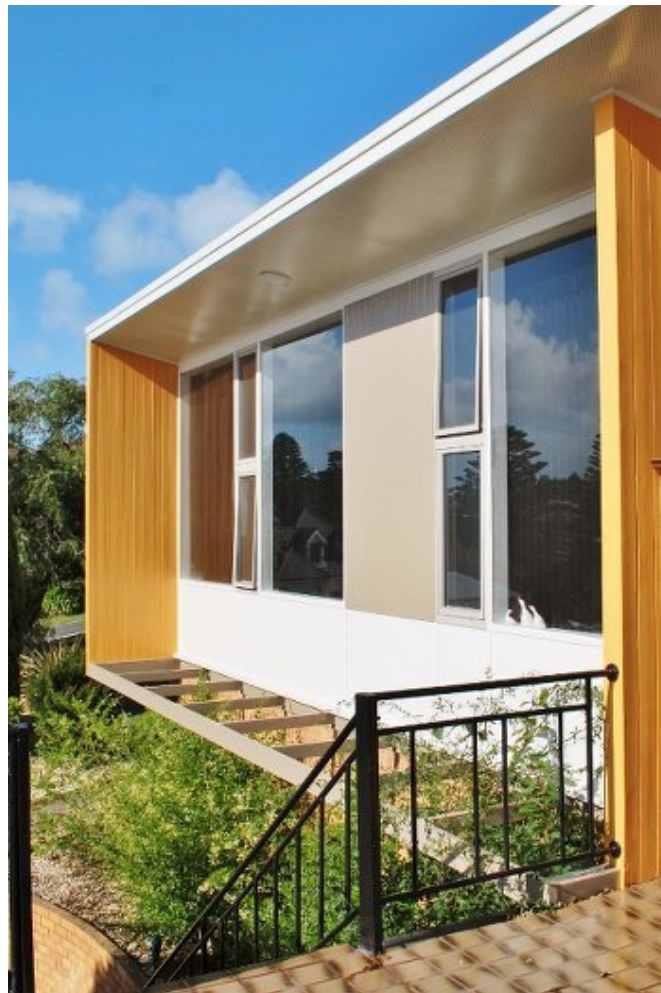
Geometric windows, brightly coloured blade walls and a soaring roofline add drama and excitement to the main façade. Image: Clinton Krause.
